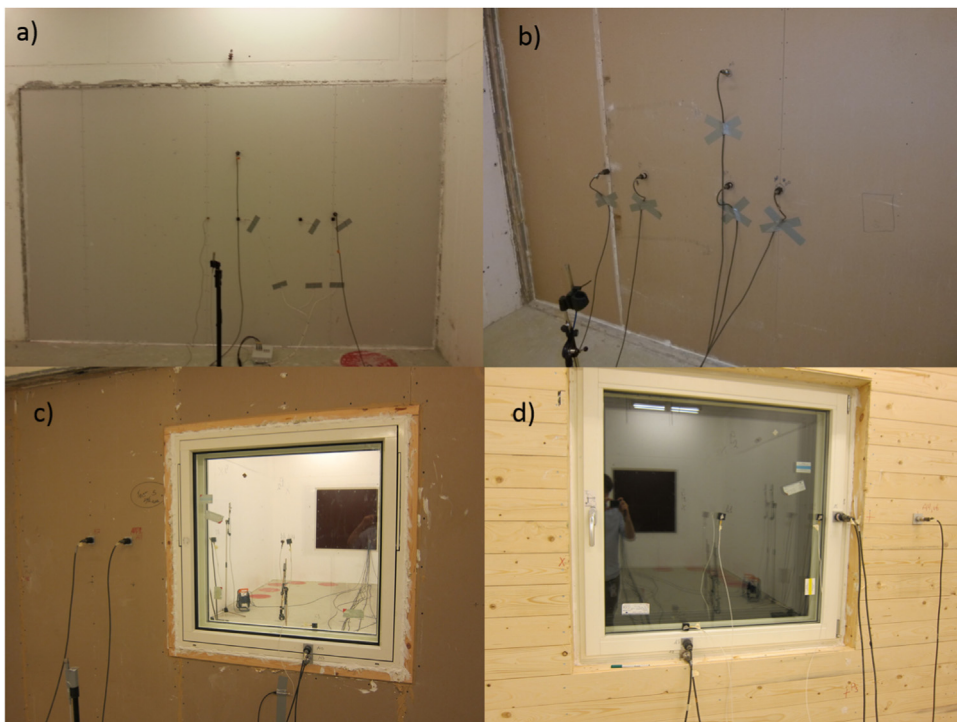
Fig. 4. Photographs of the wall and window instrumentation. (a) shows the accelerometer positions in the source room for the standard wall (S), (b) shows the accelerometer positions in the receiver room for the improved wall (I), (c) shows the accelerometer positions in the source room for a wall with window, (d) shows the accelerometer positions in the receiver room for a wall with window.
