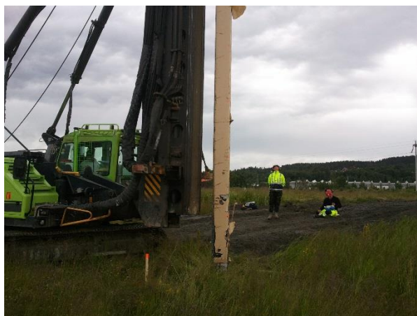
Figure 7: Test piling with PDA-testing
