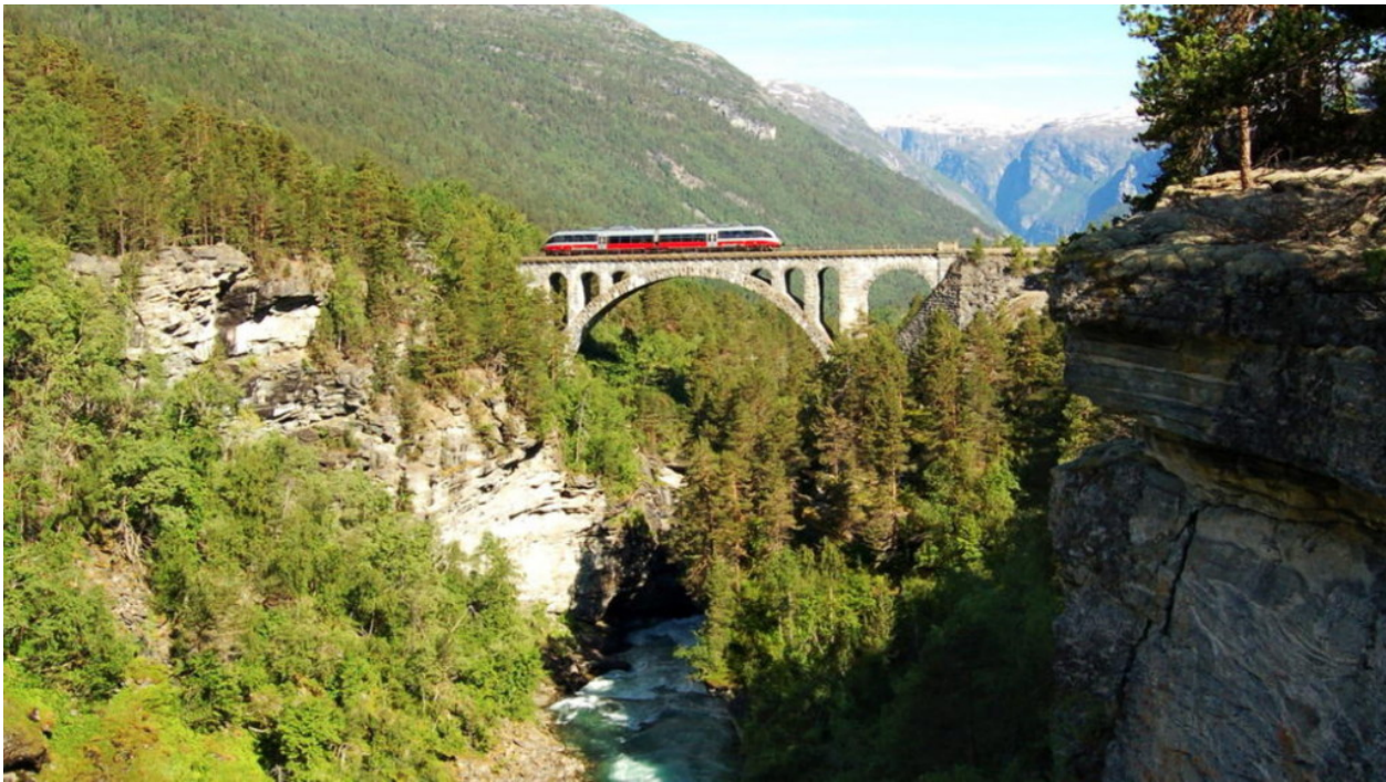
Figure 3: Kylling Bridge with a single type 93 passenger service between Dombås and Åndalsnes. The bridge is part of the second horseshoe turn at Verma.
