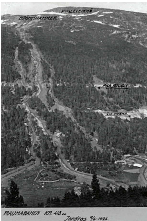
Figure 1: On the 9th of June 1926 a major landslide hit the Rauma line by Verma station. The landslide crossed the line twice, on both sides of the horseshoe turn in "Vendetunellen"
