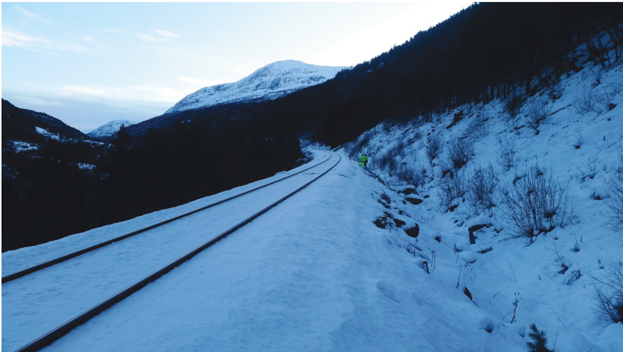
Figure 5: The line below Rensken. Several rocks and boulders can be observed partially covered by the snow beside the track. The photo was taken on the 27th of November 2017 during the installation of the sensor units.
