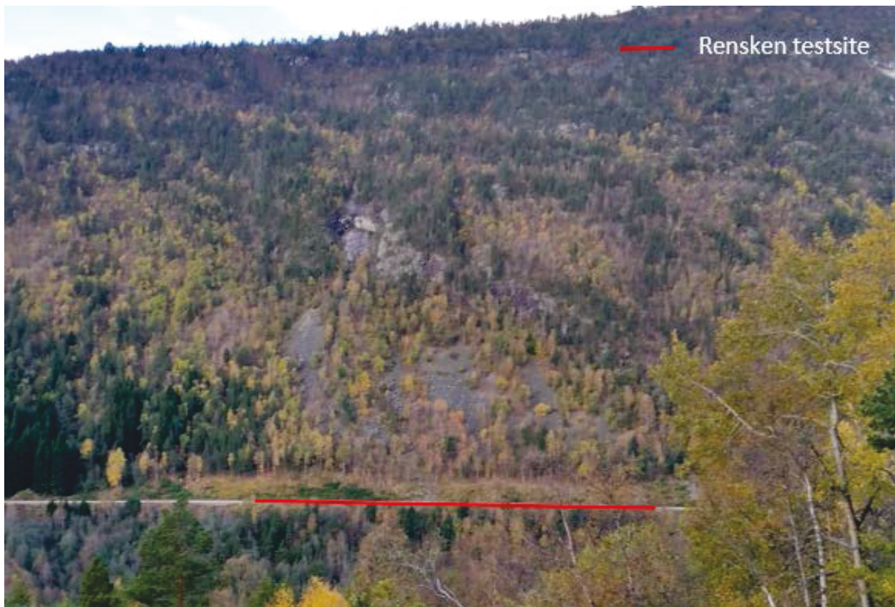
Figure 2: The GoSafeRail test site for rockfall and landslide detection cover a 330 meter long section of the Rauma line. The cliff directly above the line is named "Rensken", implying that considerable effort was made to clear the area of loose rocks when the line was built. Observations indicate that there are rockfalls annually on the site.
