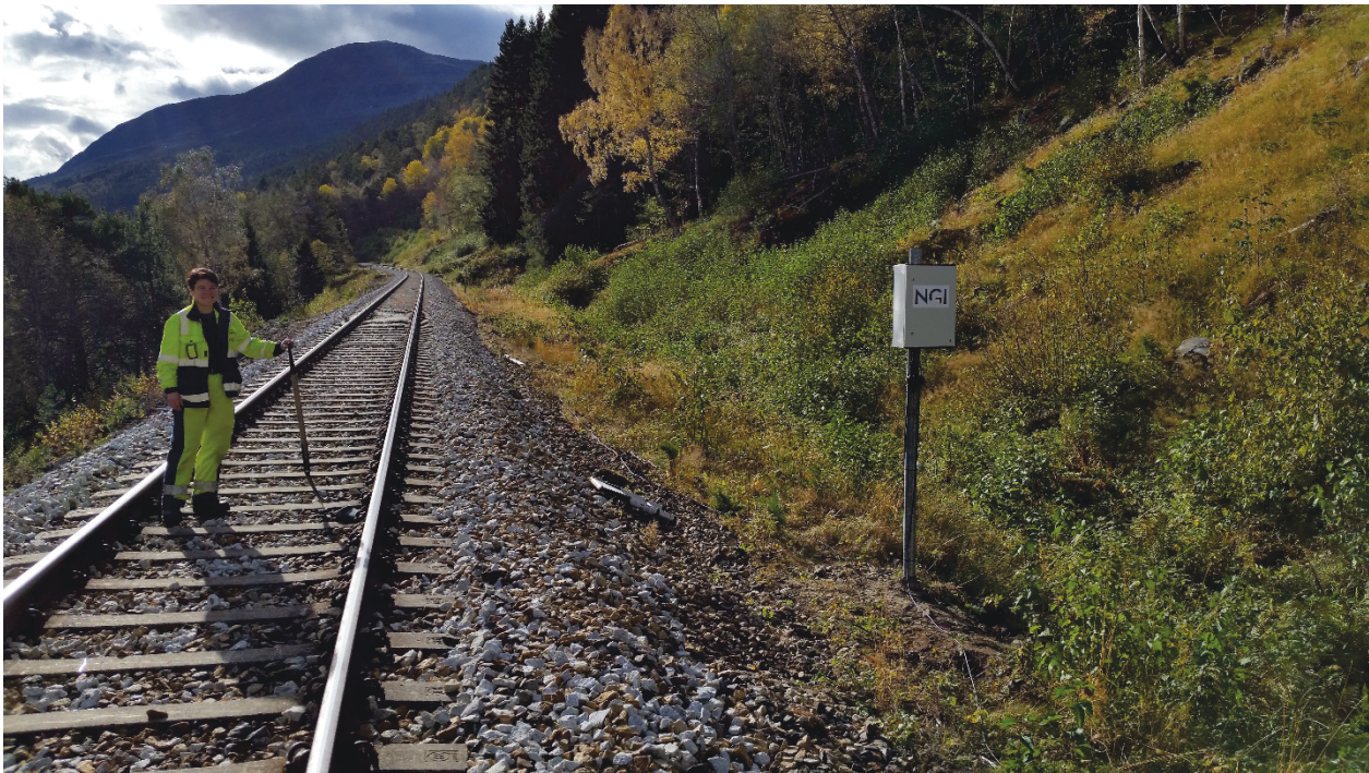
Figure 8: A second electronics cabinet is installed next to the line at the test site. This contains two relay radio units with directional yagi antennas. One antenna is directed towards the gateway on the opposite side of the valley, while the other is pointing towards the sensor units in the track. For optimal protection during snow moving, both antennas are mounted inside the enclosure.
