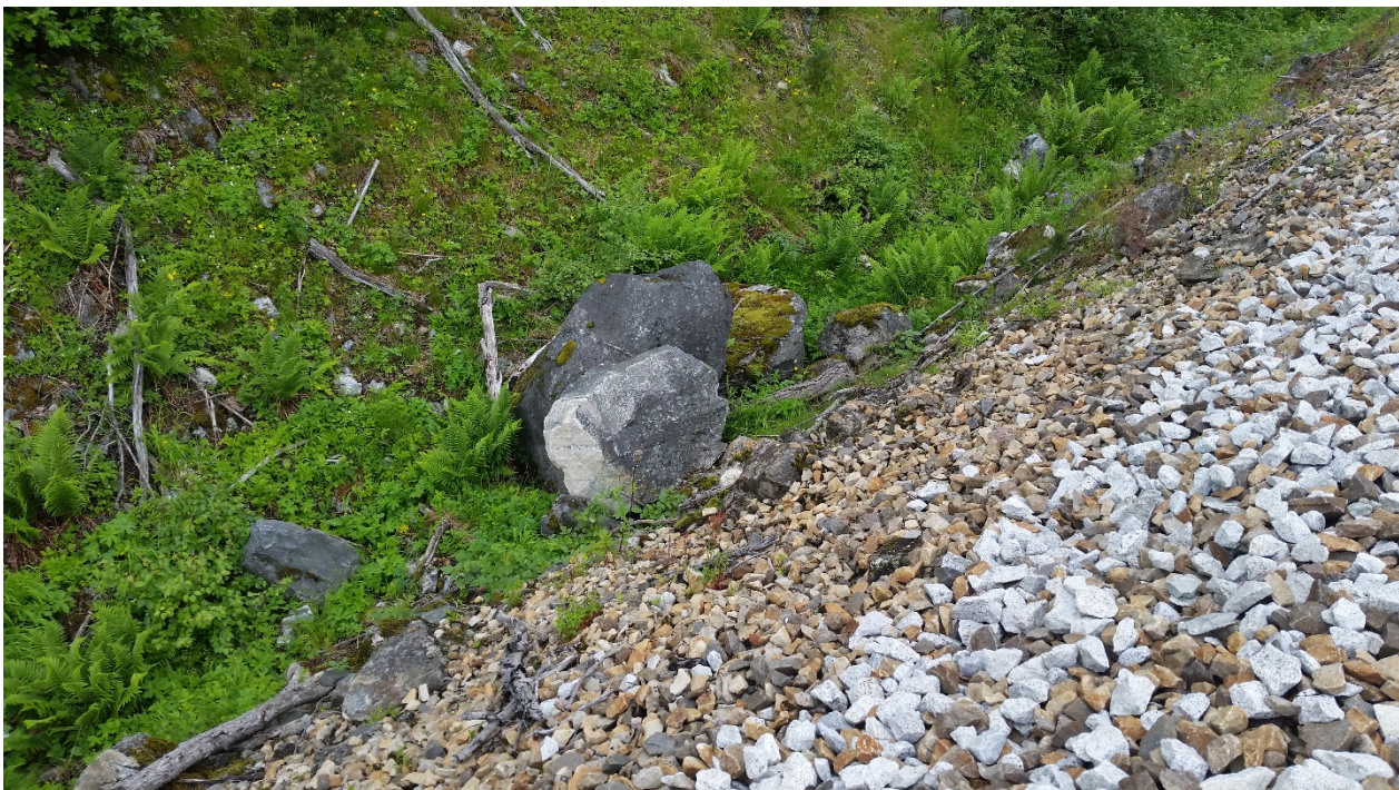
Figure 9: A single rockfall will generate a shockwave in the track, propagating in both directions from the point of impact. This acoustic signature is distinguishable from most other events, when the shockwave is strong enough to be detected by several sensors on both sides.
