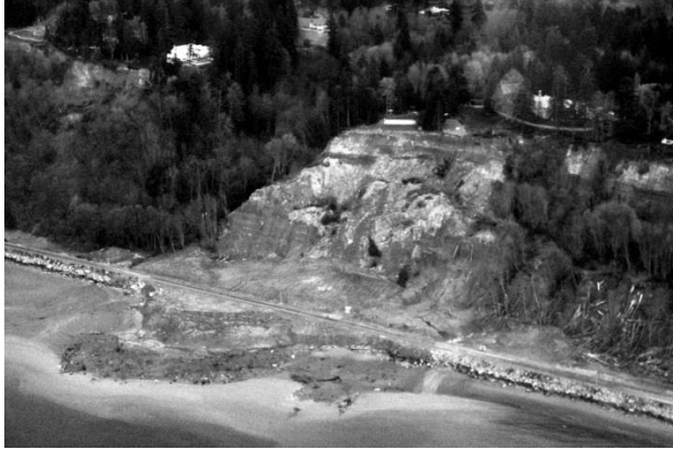
Figure 4. Photo of 15 January 1997 Woodway landslide (courtesy of H. Shipman).
