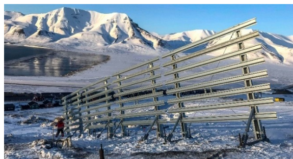
Figure 7. Snow fence under construction spring 2018. Photo: Eli Margrethe Solberg.
