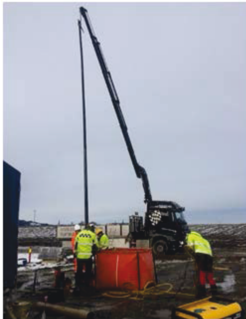
Figure 27. Installation of soil freezing pipes at Øysand in March 2019.
