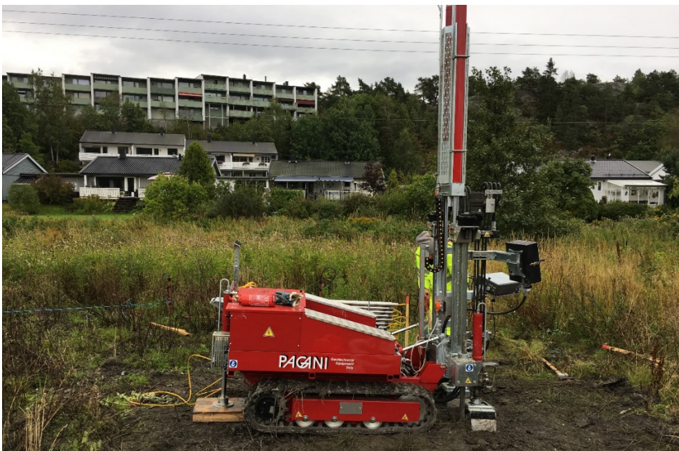
Figure 4.7.2 Pagni rig used for cone penetration testing
