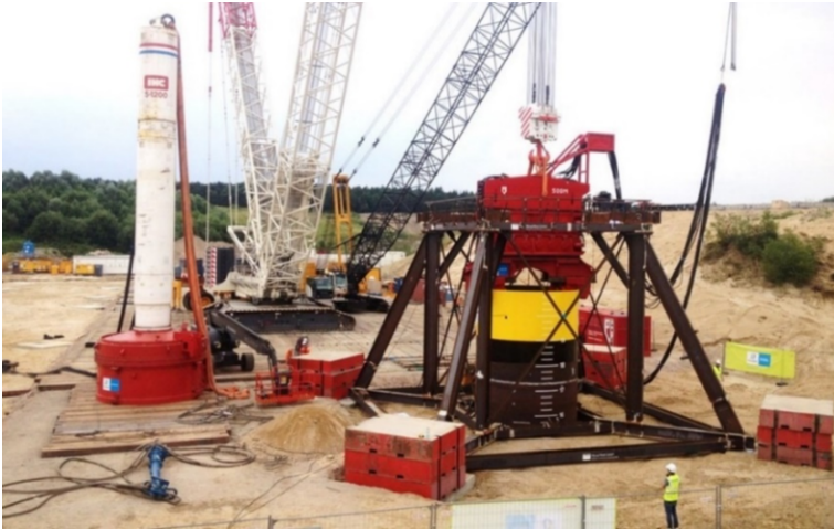
Figure 27. Vibro test in Cuxhaven (Germany), Photo: RWE.
