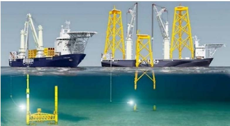
Figure 28. Pile driving using seabed template and subsequent jacket installation (Illustration: Jumbo shipping).
