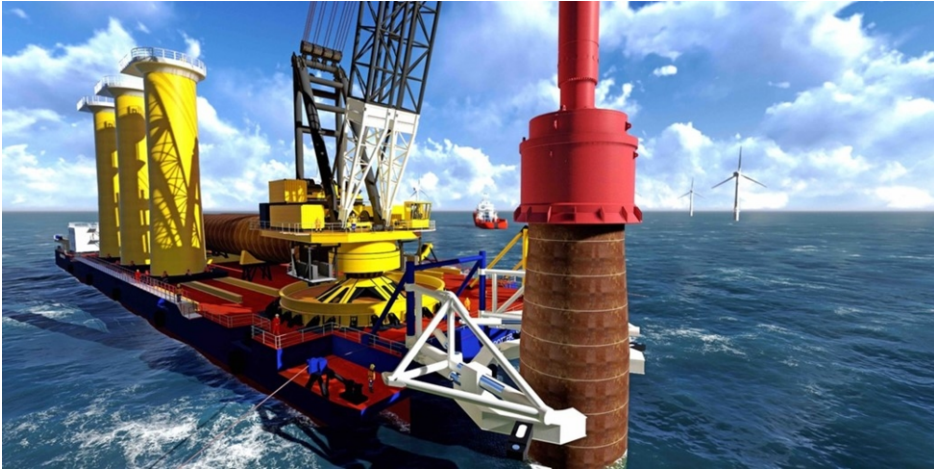
Figure 25. Monopile driving from a floating vessel with motion compensated pile grippers for control of the pile verticality. The transition pieces are installed after completed pile driving and stored upright on deck to the left in the picture (Illustration: Quest Offshore).
