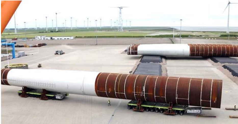
Figure 18. The world's largest monopiles produced by EEW 2016 for the German "Veja Mate" wind farm, total weight 1 300 tons, 7.8m diameter at mudline and 82m long.
