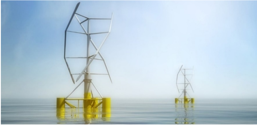
Figure 36. Floating deep-water foundations with Vertical Axis Wind Turbines (VAWT's), Image: InFLOW.
