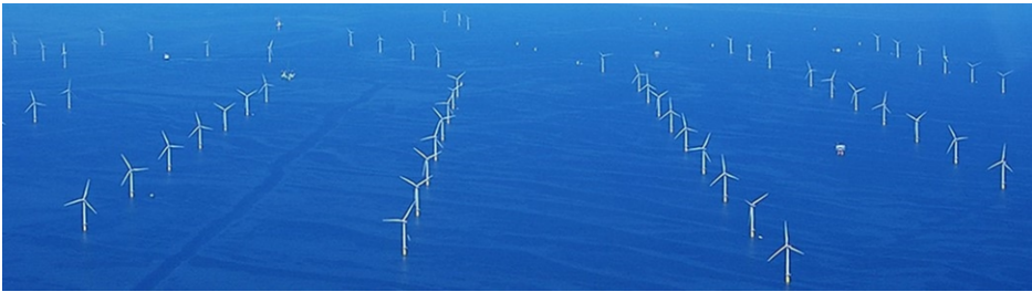
Figure 2. The Walney Wind Farm operated by Ørsted in the Irish Sea is presently (2018) the world's largest operating offshore wind farm with 189 OWT's producing 659 MW of power (photo: Ørsted).
