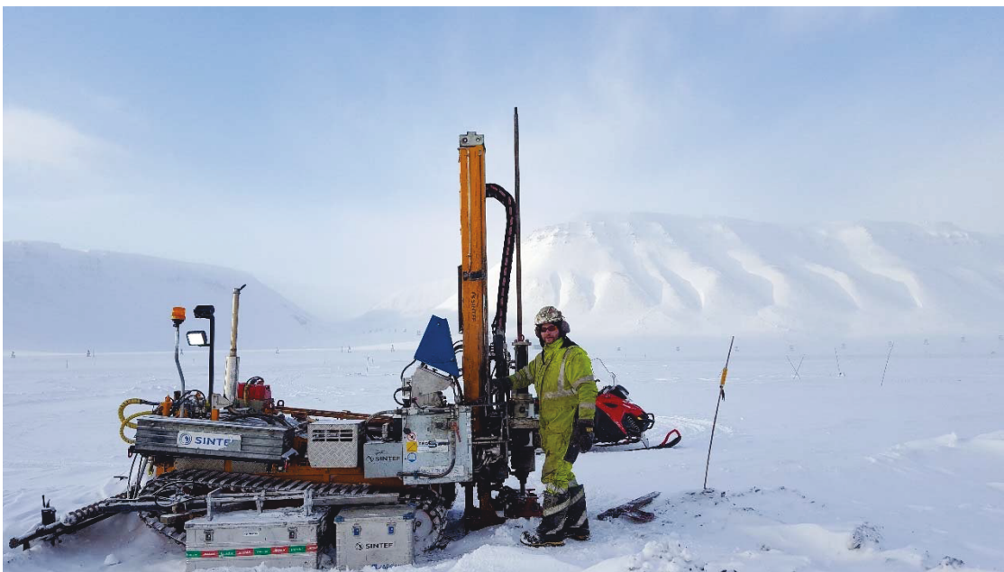
Figure 4 The SINTEF drilling rig in operation in Adventdalen.
