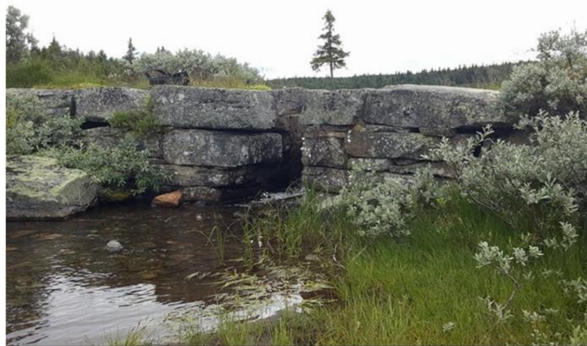
Figure 5. The old (>100 years) dam in the catchment of river Skurdalsåa (Location G2 in Figure 3). The height of the dam will be increased by 0.5–1.0 m, but the appearance will remain (photo: “Skurdalsåas venner”).
