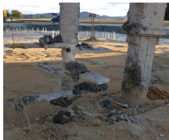
Figure 3. Mixing tool used for installation of lime-cement piles
