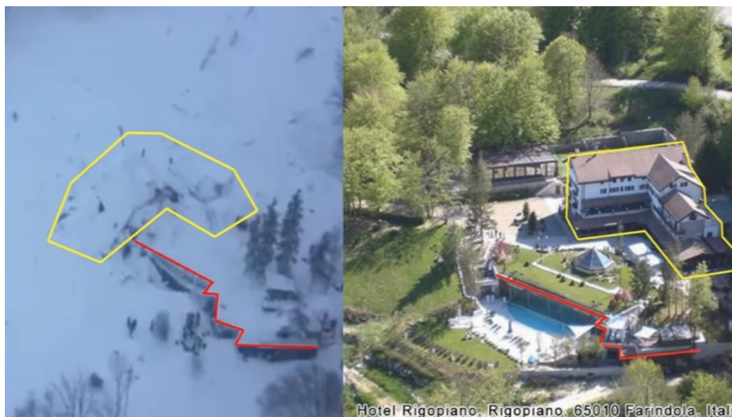
Figure 9. Position of the destroyed Hotel Rigopiano (yellow lines) before ( right panel ) and after the avalanche ( left panel ) relative to the structurally stable edge of the spa area (red lines). Still image downloaded from [11] and reproduced under Creative Commons license CC-BY 3.0, extracted from Youtube video uploaded by TvSEI ( https://www.youtube.com/watch?v=6La91fbpbbg ).
