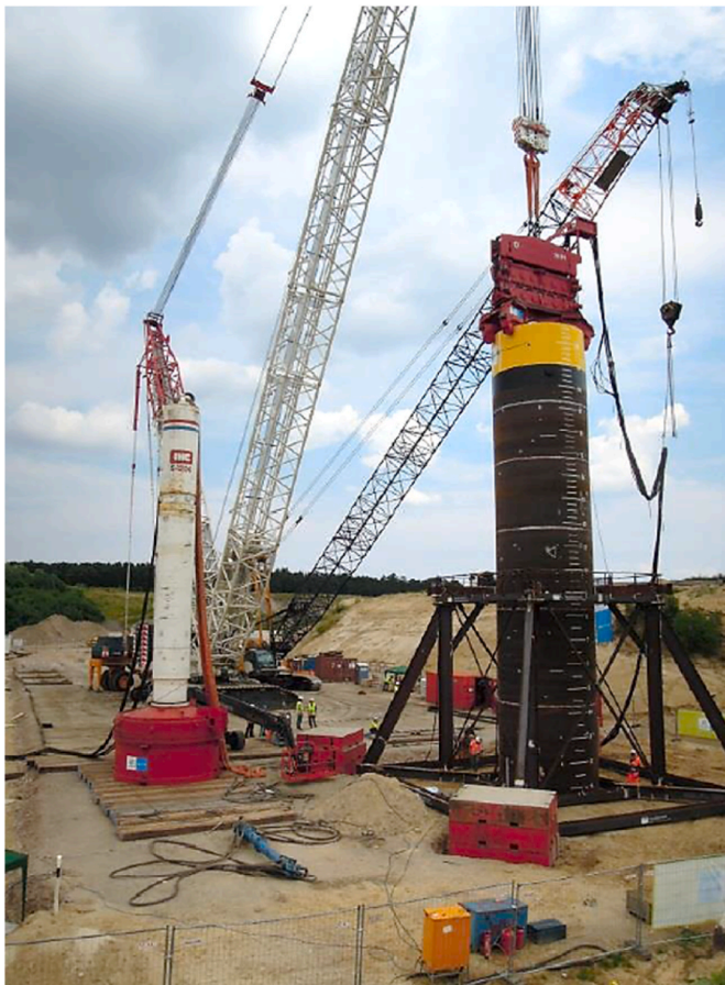
Fig. 2. Pile driving by vibration at Altenwalde [17].
