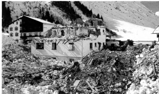
Figure 3: A building destroyed by the Galtuer avalanche (Photo: WLV Tyrol).
