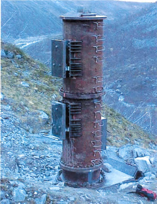
Figure 3.1.5 The steel mast with 2 load plates
