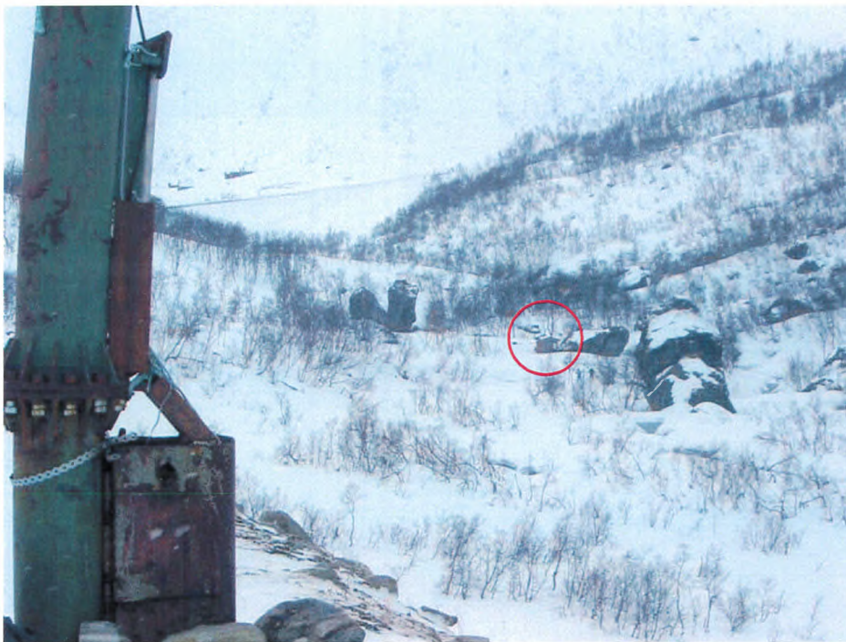
Figure 3.1.10 Instrument shelter (red circle) seen from the dam crest
