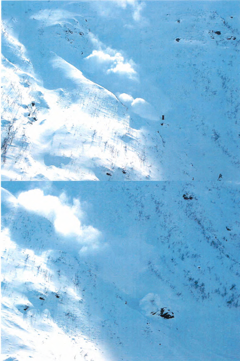
Figure 4.1.11. Impact of the April 6th avalanche on the steel tower (top) and the concrete structure (bottom).
