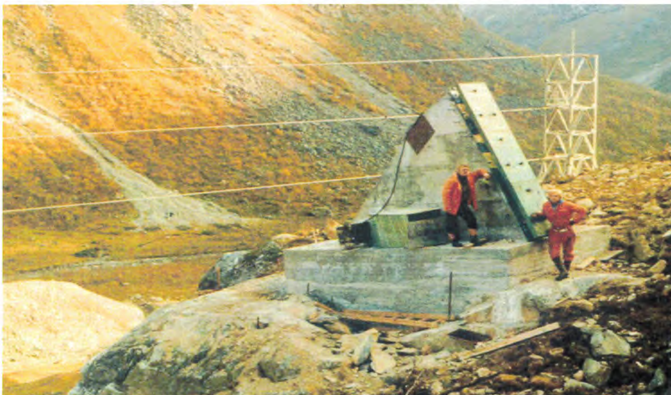
Figure 3.1.4. The concrete structure with 3 load plates
