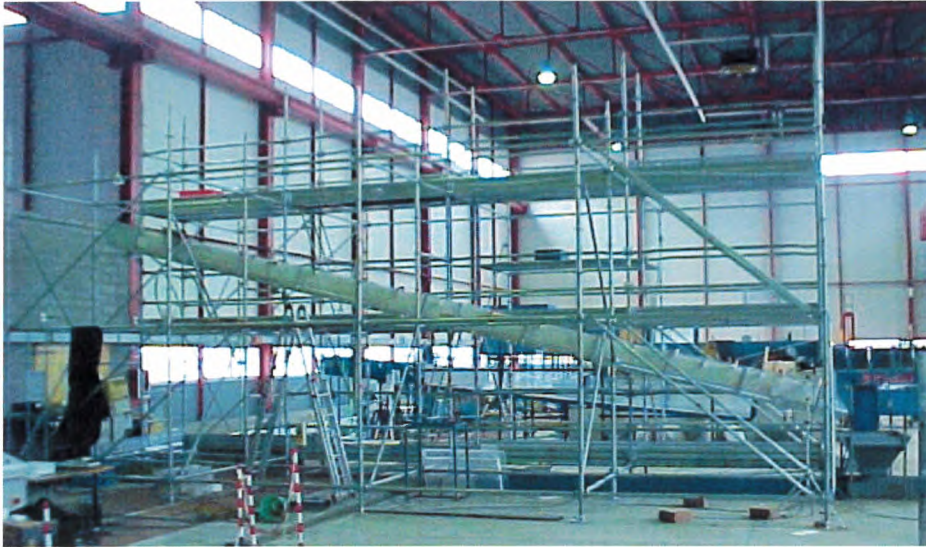
Figure 3.4.3 Side view of the Chute B and the supporting structure
