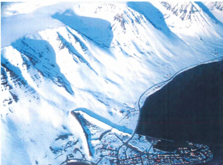
Figure 4.2.3. The deflecting wall at Flateyri, Iceland.
