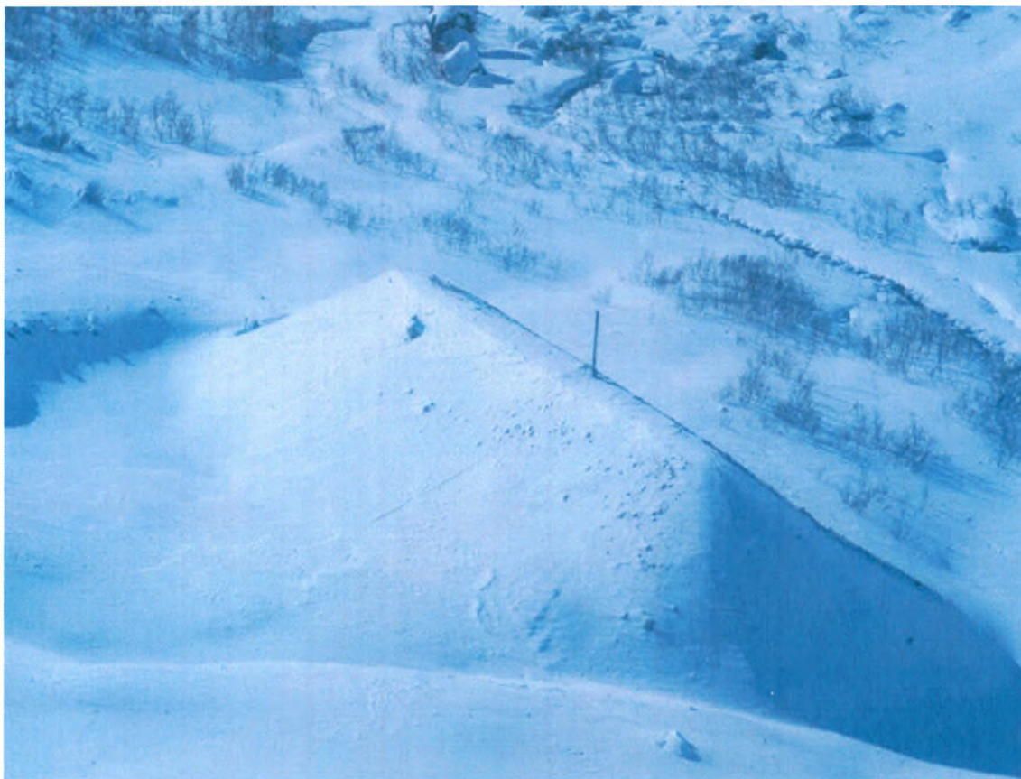
Figure 3.1.2. The catching dam with the steel mast on top
