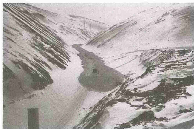
Fig. 4 Permanent slushflow hazard mitigation. Removal of snow from the potential starting zone and track in Vannledningselva, Longyearbyen, Svalbard, is done every spring to protect the development area on the fan. The large rockfill in the right half of the picture is part of the old direction control work. (Photo E. Hestnes, NGI)
