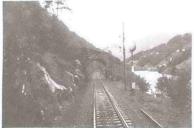
Fig. 9 A small shed specifically built for protection against slushflows. Bergen-Voss railway, West Norway. (Photo E. Hestnes, NGI)
