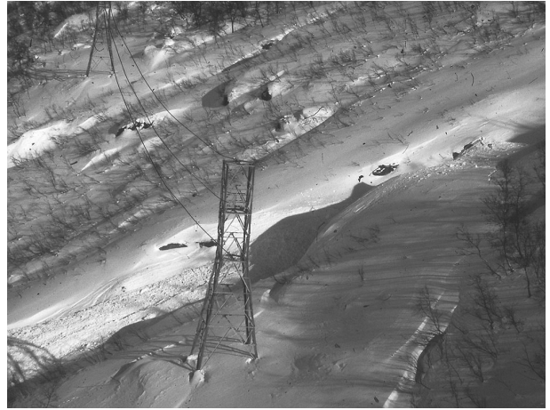
Figure 10: Transmission line assembly (photo NGI).
