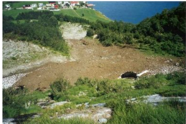
Figure 3: Indre Standal, Ørsta municipality. The upper deflecting dam (“Standal Fortress”) is partly visible at the left edge of the picture. The outer curve of the lower deflecting dam appears as a bright area in the middle upper part of the picture (from SW).
