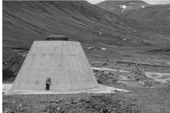
Figure 3. Foundation of one of the Y-towers in Áreyjadalur. The view is up the valley; the foundations of other towers in both of the lines can be seen. The kid leaning at the foundation is about 1.1 m tall. Photo: Árni Jónsson 16/7 2006.
