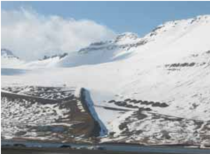
Figure 15.1: Deflecting dam and braking mounds at Seljalandsmúli in Ísafjörður, northwestern Iceland. The dam is 650 m long and 16 m high, and the braking mounds are 7 m high. The total volume of fill material in the dam and mounds is 360,000 m 3 . (Photo: Tómas Jóhannesson.)
