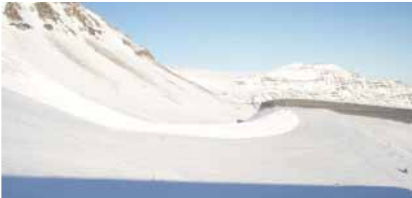
Figure 3.2: A catching dam at Brún in Bjólfur in Seyðisfjörður, eastern Iceland. An avalanche that fell on 9 February 2008 and stopped just at the dam face can be seen. The dam is 20 m high with a 10 m high very steep upper part. (Photo: Emil Tómasson.)
