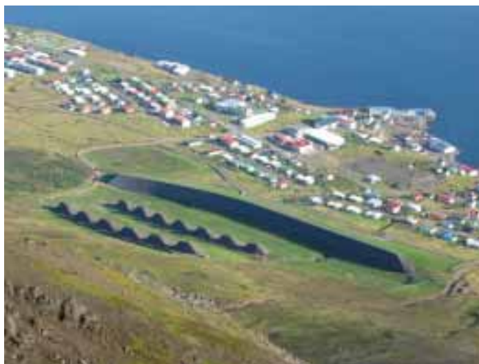
Figure D2: The braking mounds at Neskaupstaður and the catching dam behind them. Each mound is 10 m high and the catching dam is 17 m high. (Photo: Tómas Jóhannesson.)
