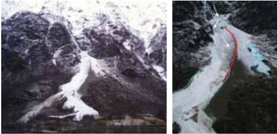
Figure C5: Deflecting dam at Langageiti, western Norway, after the second avalanche during the winter 1998/99 (photos: NGI). The second avalanche overtopped the lower part of the dam. The first avalanche overtopped the uppermost part of the dam. Arrows on the photo to the right show the assumed flow direction of the second avalanche; the red curve shows the outer extension of the flow, the dotted blue curve shows the outer extension of the deposits; the light blue area shows deposits of the first avalanche.
