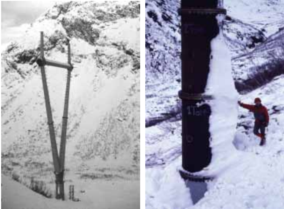
Figure 12.1: A mast built for studying impact forces on electrical power lines (left), and an instrument tower (right) that has just been hit by an avalanche in the Ryggfonn avalanche path in western Norway. The power line mast was broken several times by avalanches during the investigation period. (Photos: NGL.)
