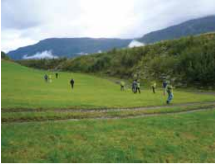
Figure 15.5: A catching dam for wet snow avalanches and debris flows. Dry wall with backfill of earth materials, height 12 m, inclination 1:1. Ullensvang, Norway. (Photo: Karstein Lied.)
