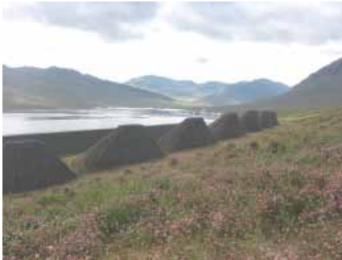
Figure 15.8: A row of 10 m high braking mounds at Neskaupstaður (see map in Fig. 15.7) (photo: Tómas Jóhannesson).
