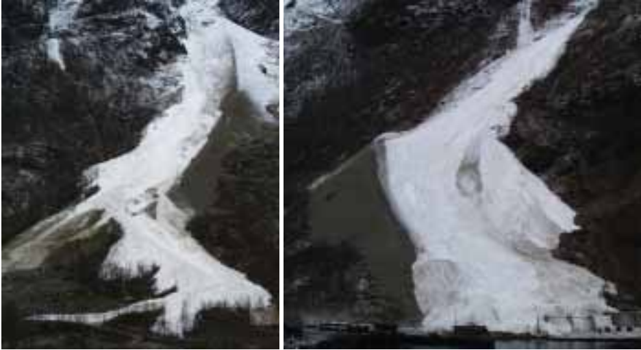
Figure 8.4: Several wet-snow avalanches may fill up the storage capacity for a deflecting channel even in fairly steep terrain as shown here for deflecting dams at Langageiti (left) and Nautagrovi (right) in western Norway (photos: NGI). The figure from Langageiti shows how a part of an avalanche may turn sideways after the avalanche overtops or flows past the downstream end of a deflecting dam.
