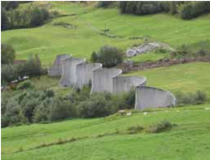
Figure 15.11: A retaining dam made of six 20 m wide and 10 m high reinforced concrete shells at Ullensvang, Norway (designed by NGI and Instanes AS, Norway). Maximum design avalanche impact force is 92 kPa. Each shell has four vertical steel anchors, each with a capacity of 2800 kN, drilled 12–14 m into the bedrock. Tilting moment on each shell is 59,000 kNm, and shear force is 8500 kN. (Photo: Ulrik Domaas.)
