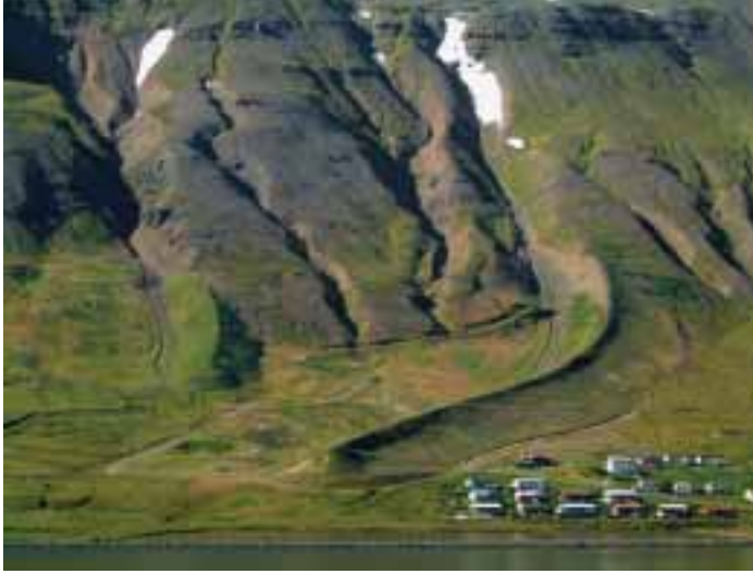
Figure C2: Deflecting dams at Siglufjörður, northern Iceland. The larger Strengsgil dam is 18 m high and the smaller Jörundarskál dam is 15 m high. (Photo: Reynir Vilhjálmsson.)
