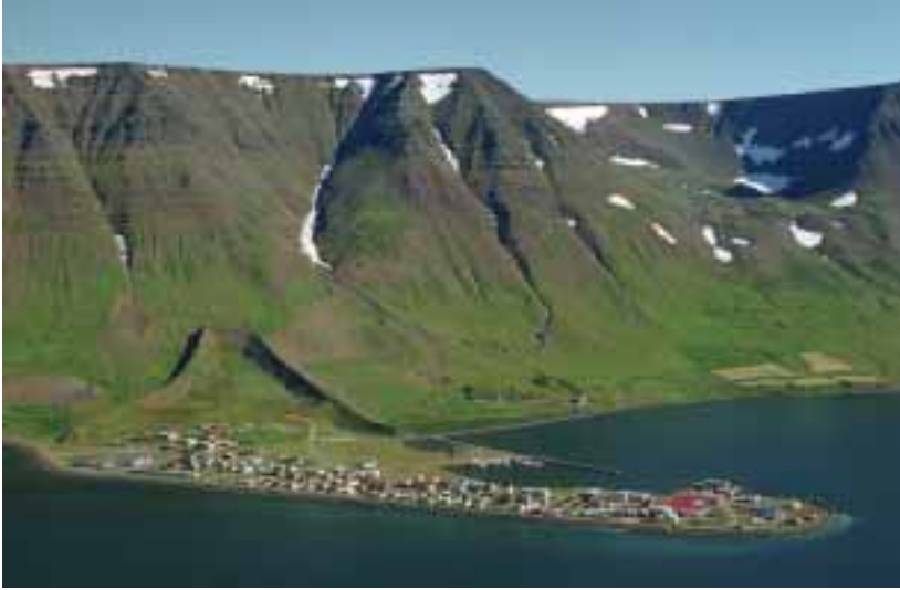
Figure 3.3: Two deflecting dams and a catching dam at Flateyri, northwestern Iceland. The deflecting dams are 15–20 m high and the small catching dam between them is 10 m high. The dams were built after a catastrophic avalanche in 1995 that killed 20 people. (Photo: © Mats Wibe Lund.)
