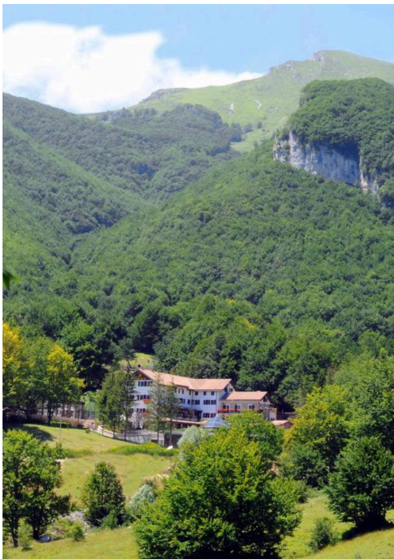
Figure 5 View of the hotel before the 2017 avalanche. The original cabin Rifugio Tito Acerbo (small grey stone structure to the right) was integrated into the much larger new building. Note the dense forest along the avalanche track. Image from the website https://geograficamente.wordpress.com/2017/01/30/il-duro-inverno-dellappennino-centrale-terremoto-neve-valanghe-e-impreparazione-agli-eventi-naturali-in-mano-alleroismo-di-pochi-il-caso-dellhotel-rigopiano-e-il-per/ , retrieved on 2017-09-01
