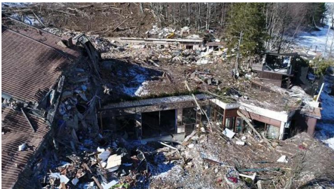
Figure 6 Partial view of the destroyed Hotel Rigopiano. The spa area in the foreground is moderately damaged, but the upper two floors of the old Rifugio Tito Acerbo were annihilated and the four-story main complex collapsed completely and was displaced by some 10 m. Photo from http://primadano.i.it , retrieved on 2017-08-09
