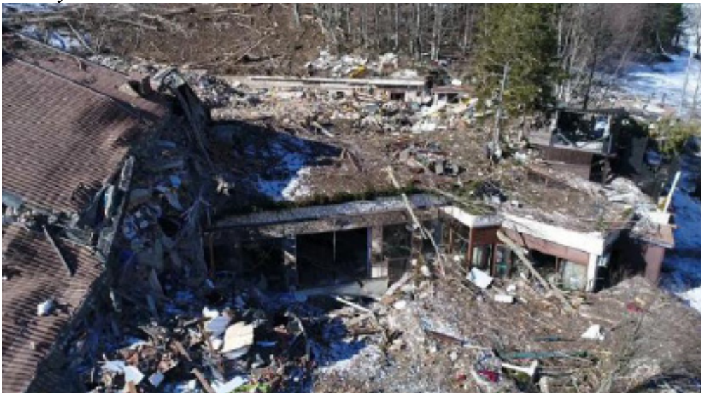
Figure 16 The destroyed main wing of the Hotel Rigopiano to the left, the spa area in the middle and the original Rifugio Tito Acerbo near the forest in the background
