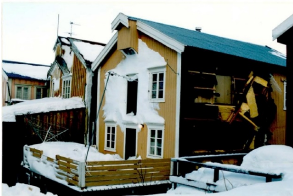
Figure 7 Signs of “air blast” impacts: right) snow deposits and damage caused by the ‘skredvind’ of the powder snow avalanche from Stortuva, Mosjøen, Norway, on 29.02.1996 (photo NGI); left). \alpha -angle of the dense part (filled marker) and for the reach of powder part of the avalanches (open marker) versus the \beta -angle. The dashed line shows the fit angle \bar{\alpha}(\beta) = 0.96\beta - 1.4^\circ according to (Lied and Bakkehøi, 1980) and the gray-shaded area marks the corresponding \pm 1\sigma -range
