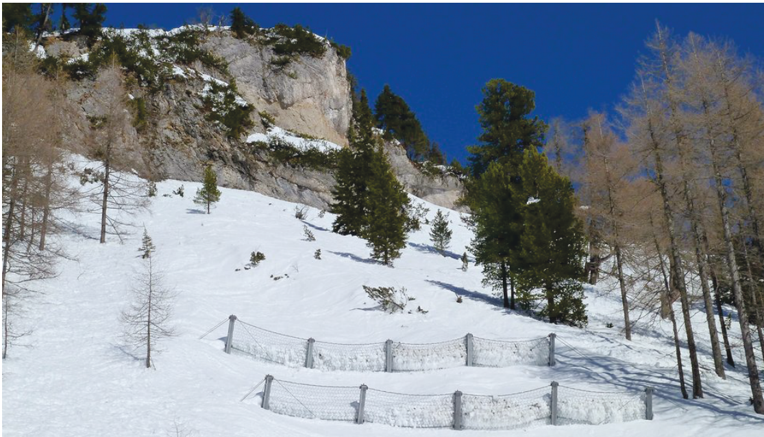
Figure 8. Steel nets for stopping a small avalanche in Austria. Image taken from the producer's website ( https://www.rud.com/en/products/barriertech/avalanche-protection.html )
