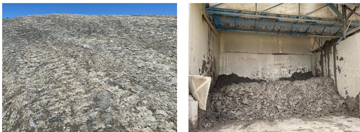
Figure 1. Excavated cement stabilised soil at immediate storage area before being used as sealing layer (left). Press filter residual (PFR) in the filter press (right).
