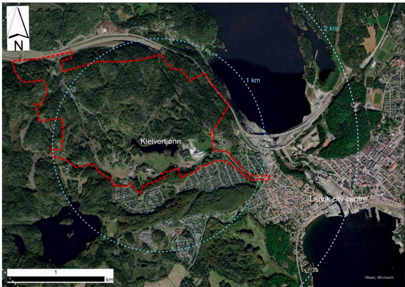
Fig. 2. Aerial photo of Larvik with the Martineåsen development project outlined by the red stippled line, lake Kleivertjønn in the centre of the image, and distance radii from Kleivertjønn marked by an inner (1 km) and outer (2 km) light-blue stippled circle, respectively. (For interpretation of the references to colour in this figure legend, the reader is referred to the web version of this article.)
