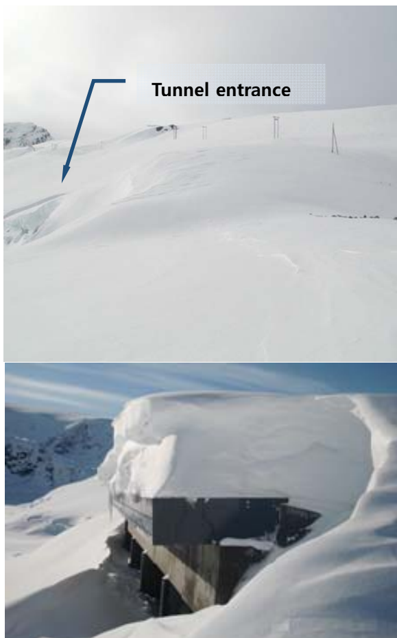
Figure 36. Approach to spillway tunnel of Dravladalen Dam in March 2000 (above) and in March 2015 (winter with heavy snow downfall (below) (Photos: Statkraft AS).
