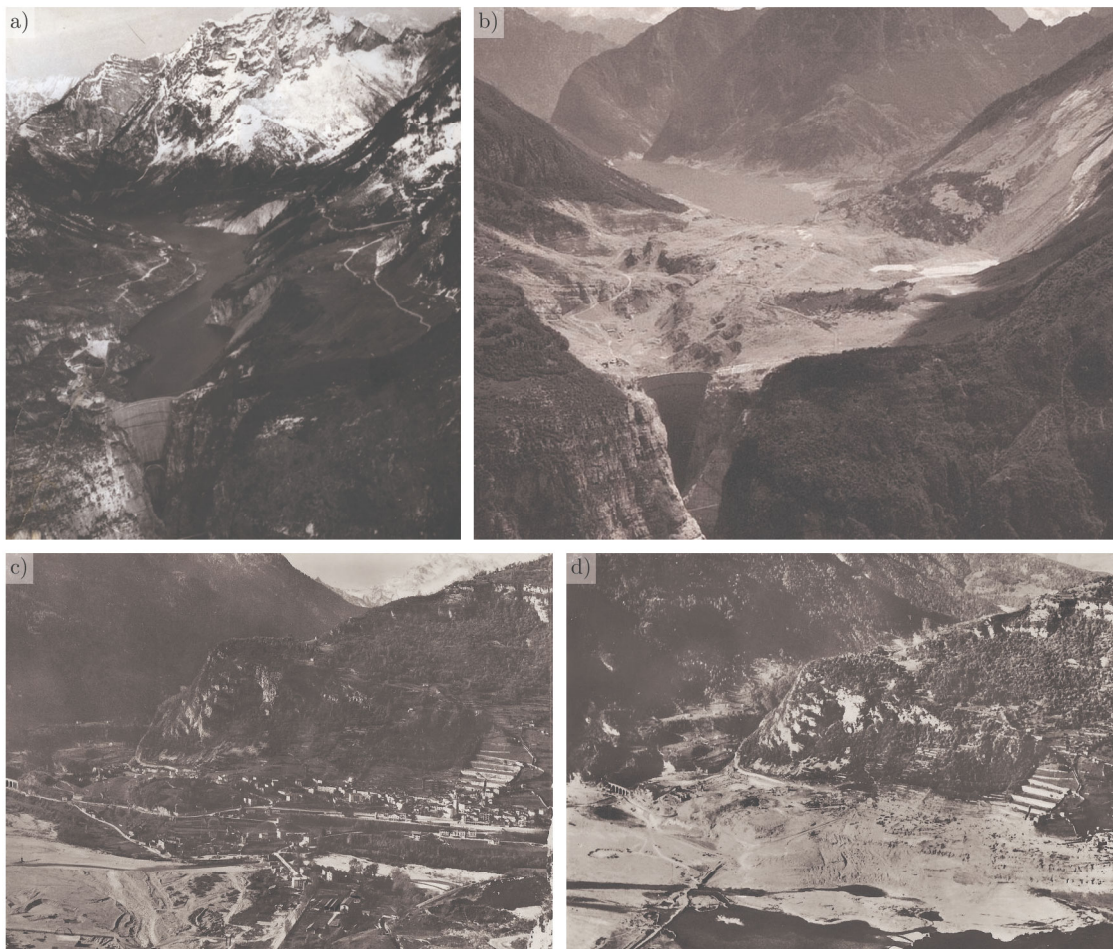
Figure 1.1: The Vajont reservoir before (a) and after the 1963 landslide (b). The landslide displaced large parts of the water and generated a tsunami that destroyed the village of Longarone, shown before (c) and after the event (d).
