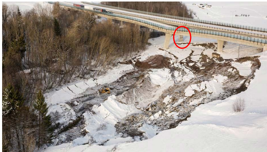
Figure 1. Quick clay landslide that caused failure of the Skjeggstad Bridge pillar. The investigated pillar, Axis 4 bridge, lies slightly outside the failure footprint and is circled in the figure (Photo: SVV 2015)
