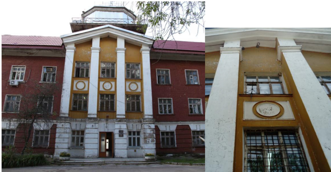
Fig. 3. left: Measurement building with measurement room in second floor, right: detail of heavy façade (facing north-west) with outdoor microphone position used during flight 1-2 in the 2019 flight campaign.
