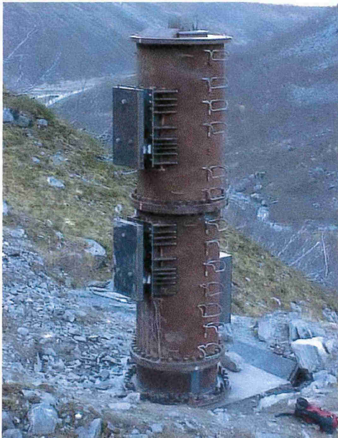
Figure 6 The steel mast
