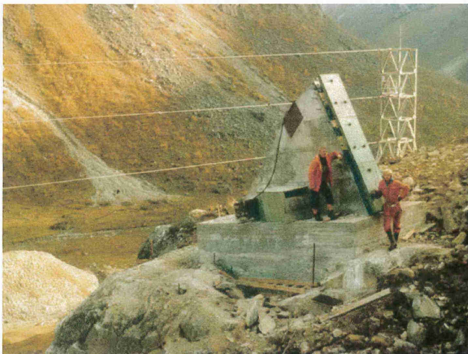
Figure 5 The concrete structure with load plates
