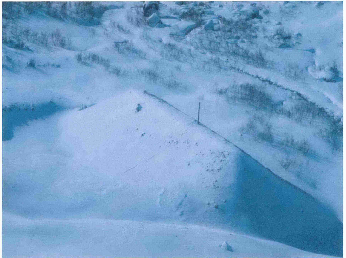
Figure 4 The catching dam with the steel mast on top
