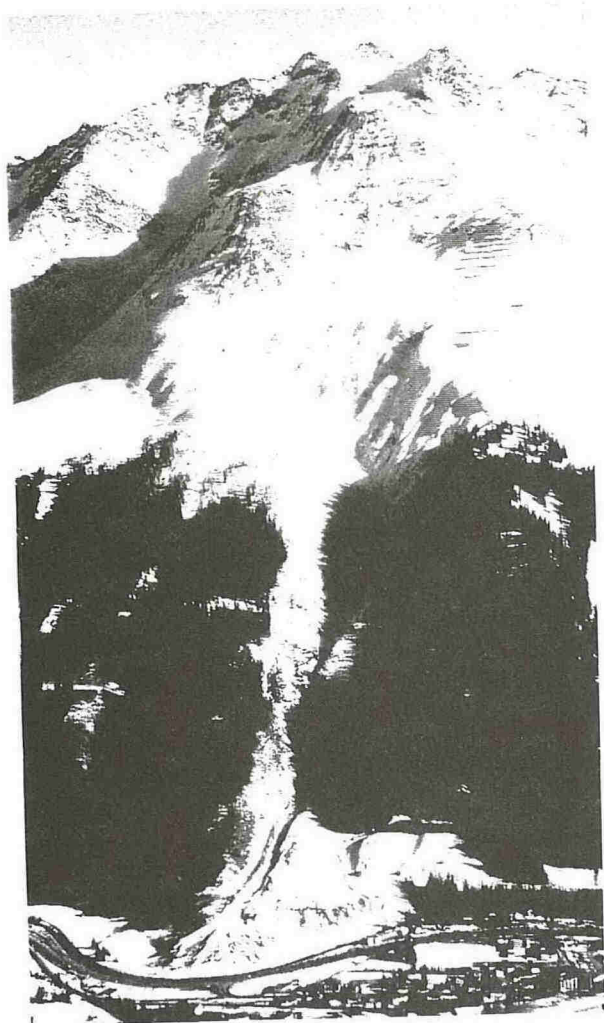
Fig. 2. Overview of the Wolfsgruben Avalanche as a typical alpine type of avalanche, Community of St. Anton, Austria; The right part of the starting area is already covered with supporting structures
