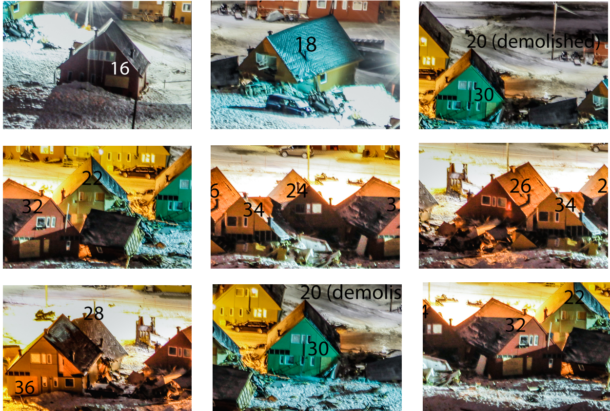
Fig. 5: Detailed views of the damaged houses (extracted from Fig. 2). The numbers correspond to those in Tbl. 2 and Fig. 2.
