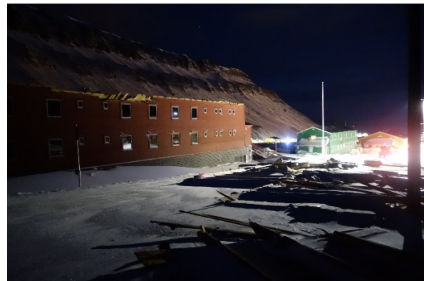
Figure 10: Roof blown of house in Nybyen. Photo: Kjetil Brattlien, NGI.
