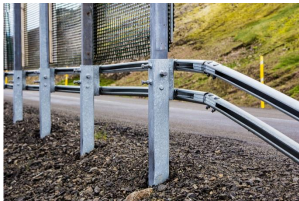
Fig. 9 A close up of one of the end posts. The guardrail end is bent down from the post into the ground.
