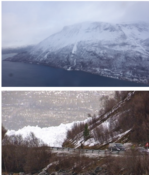
Fig. 1: Avalanche path crossing the E6 between Hatteng and Storfjord. On 11 March 2014, the road was blocked twice due to avalanches from this avalanche path. (Image courtesy: above) Kjetil Brattlien, NGI; below) Dan Henrik Klausen, NRK). This ava-
