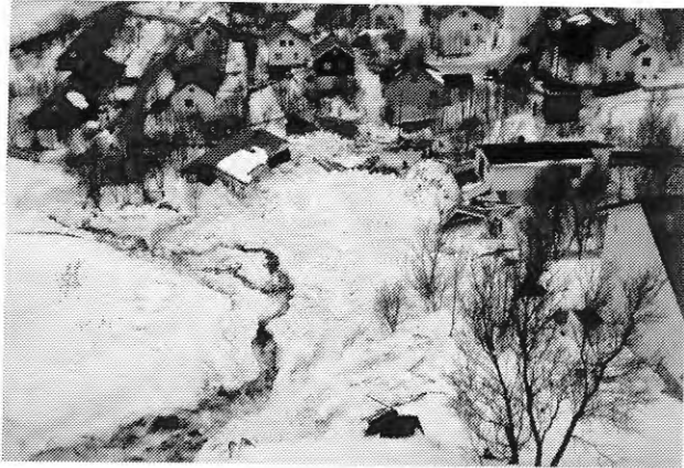
Fig. 2 A small slushflow has run into the town of Hammerfest at 71° and demolished two houses 15.02.1994. (Photo K. Lied, NGI)
