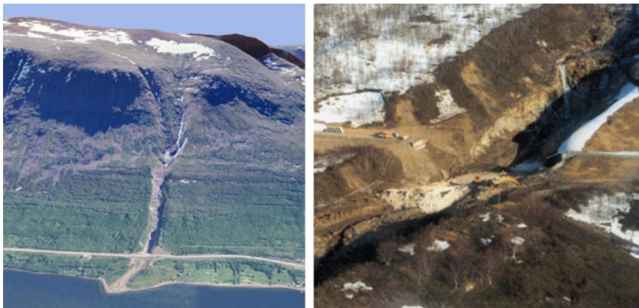
Fig. 11: Herraneselva, Langfjorden, Alta, North Norway, 19.05.2000. a) The mountainside with the two slushflow paths. Starting zones in the high-lying basins. The bridge is replaced by a fill after the bridge was lost in the fiord in 2000. ( www.kart.finn.no ) b) The crossing after the bridge was gone. It is a 800 km detour via Finland from one side to the other.
