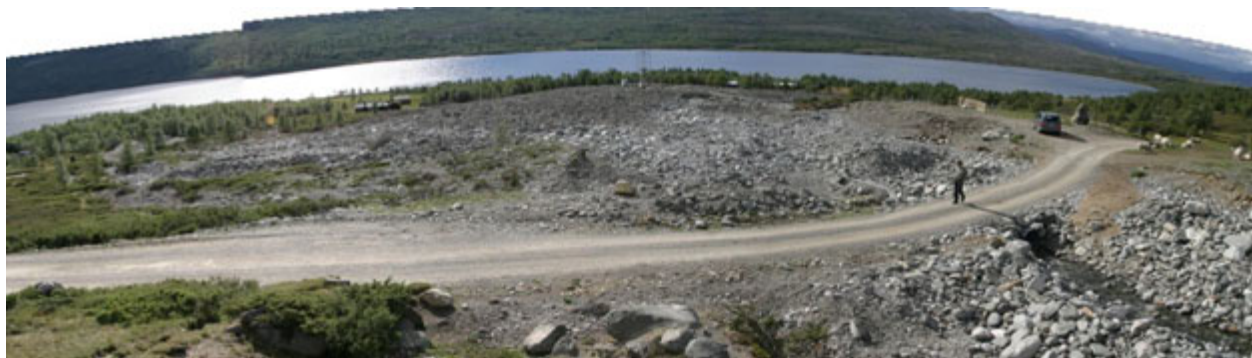
Fig. 10 Sjonsåi, Lesja, Central Norway, 06.05.2004. (Photo U. Domaas, NGI) A close up view of the deposited material documented on figure 9.
