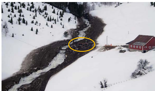
Fig. 8 Flesjaelvi, Balestrand March 21, 2011. A couple lost their lives when a house was hit by a slushflow. The house (circle) had been built without the compulsory hazard evaluation required by the Norwegian Building Code. (Photo U. Domaas, NGI)
