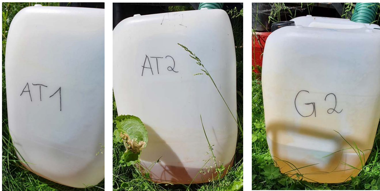
Figure 58 Iron precipitates in canisters collecting water from SVV containers AT1, AT2 and G2. (Photos taken 23.06.2021)
