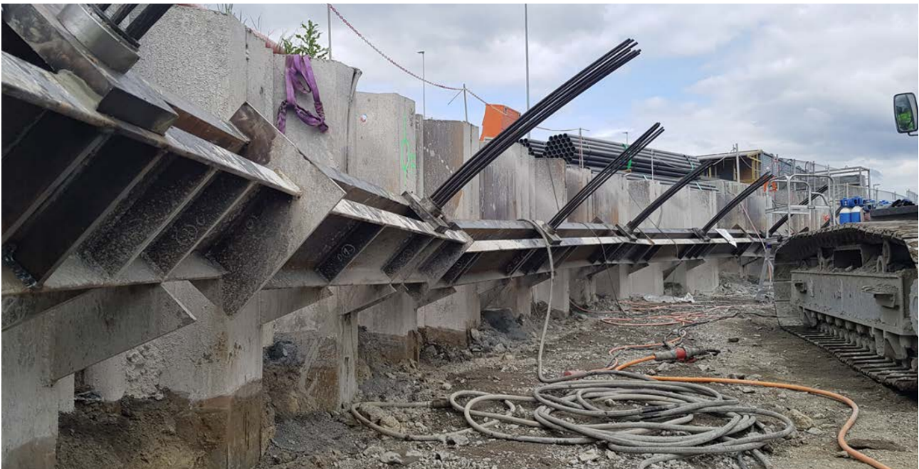
Figure 7: Simultaneous process of anchoring and excavating [11]
