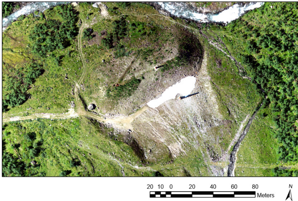
Figure 40 Drone image-derived orthomosaic of the retaining dam in summer on 08.07.2021.
