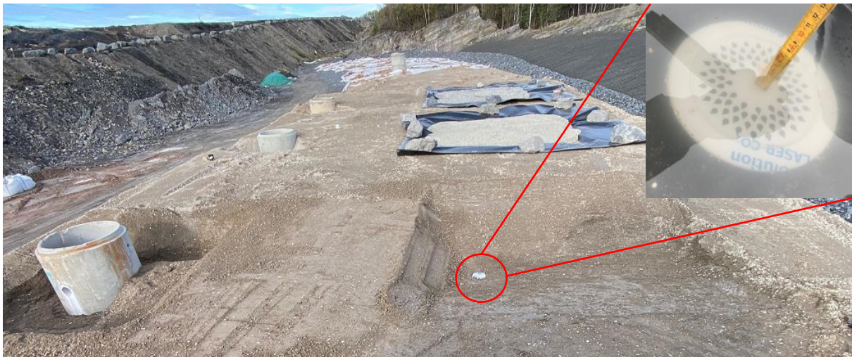
Figure 2. Construction of lysimeters. The embedded picture shows the drain during a percolation test after the geomembrane was laid out.
