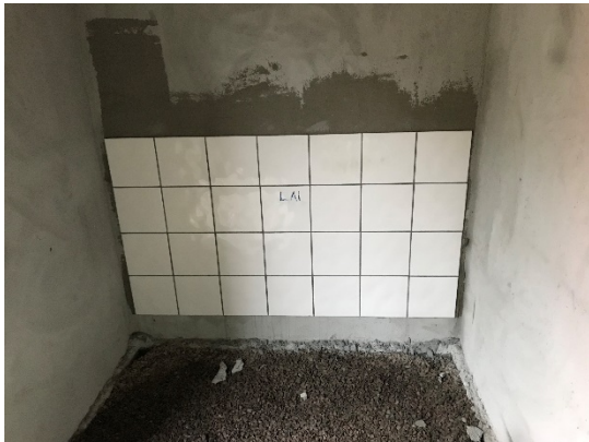
Figure 1. First blast test a) Test area (left) and test buildings (right). The casted concrete building is under construction. b) Leca building with plaster on outside. c) Inner wall of Leca building covered with tiles (the outside of this wall was facing the blasting area). d) Wooden panel mounted on one corner of the concrete building facing the blasting area.
